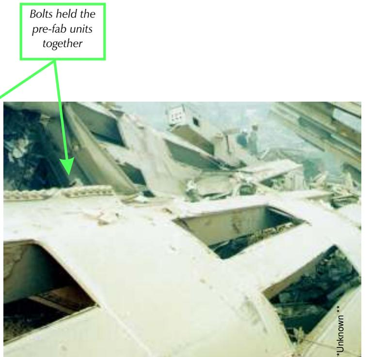
**Figure 3-11** The bolts holding the pre-fab units together.
